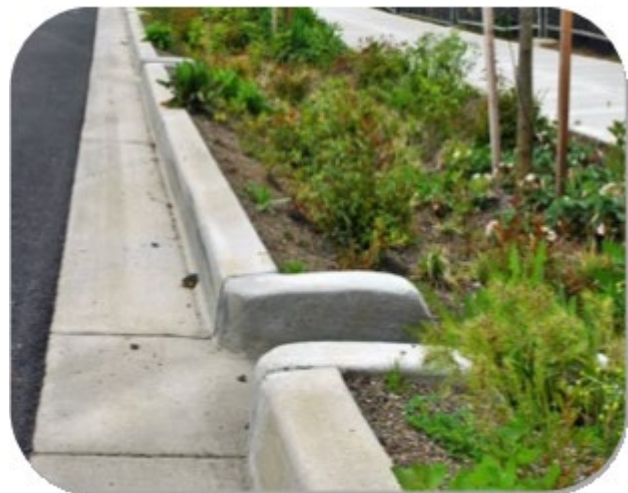
Exhibit 4.2.9D: Bioswale Curb Cut
