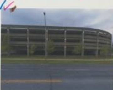
George Street Parking Garage
